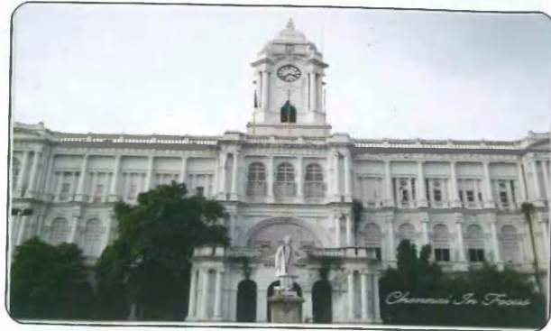
Fig. 2.42 Chennai Rippon Building
